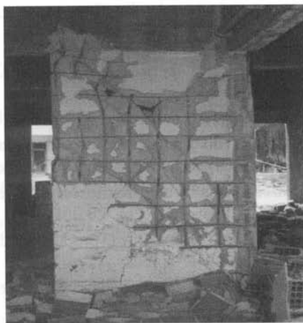
Shear wall after an earthquake.
