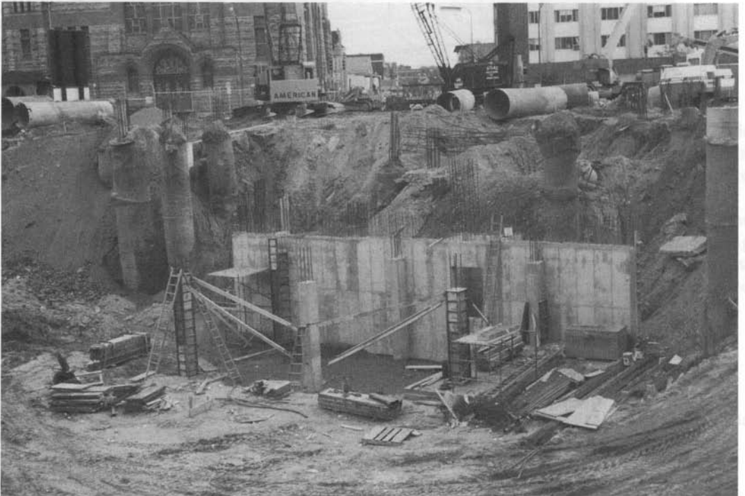
Wall and column footings, partly covered.
