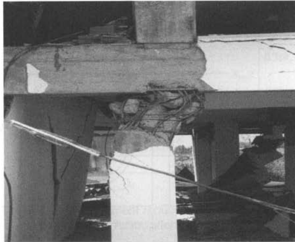
Lack of transverse reinforcement.
