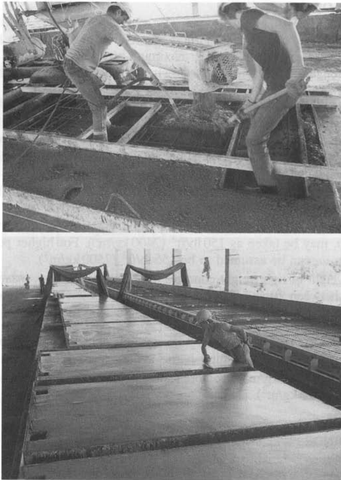
Casting and finishing precast concrete wall panels.
