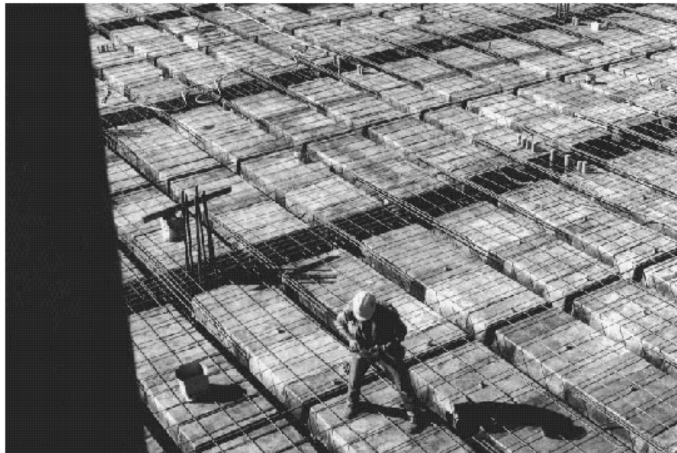
FIGURE 18.6 Steel forms for one-way joist floor.
