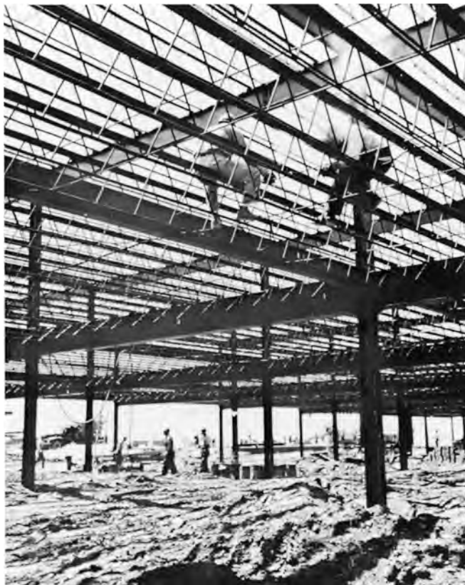
Short-span joists in the Univac Center of Sperry-Rand Corporation, Blue Bell, PA. (Courtesy of Bethlehem Steel Corporation.)
