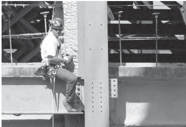
An ironworker awaits the lifting of a steel beam that will be field bolted to the column. (Courtesy of CMC South Carolina Steel.)
