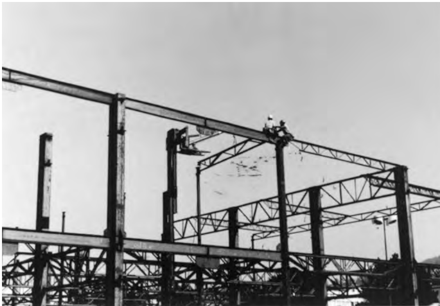
Erection of steel joists. (Courtesy of Vulcraft.)
