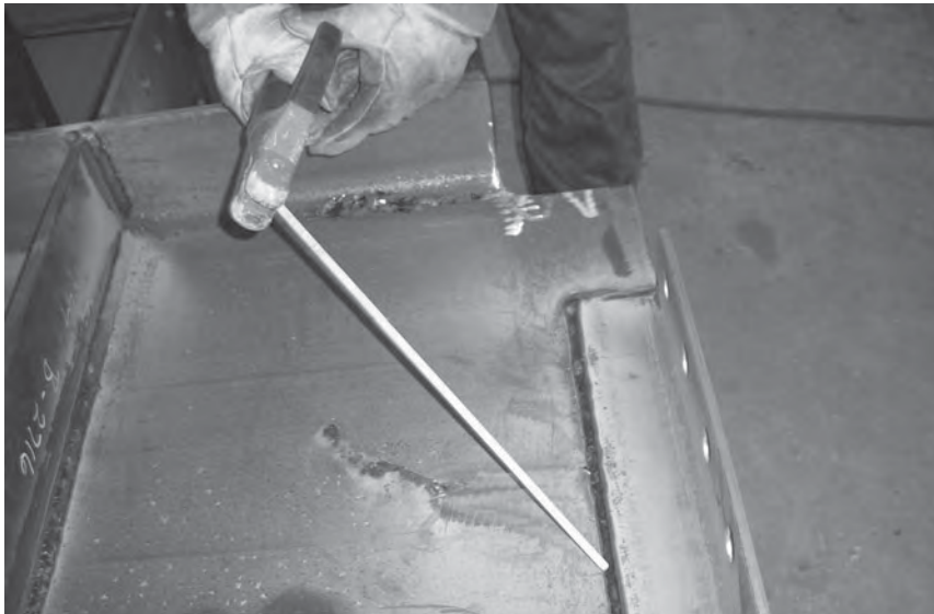
Shielded metal arc welding (SMAW) and electrode just before starting an arc to fillet weld the clip angle to the beam web. (Courtesy of CMC South Carolina Steel.)
